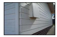
The power board should be housed within a cupboard or metal cabinet and secured with an approved electricity authority lock to restrict un-authorised tampering with the power supply.
